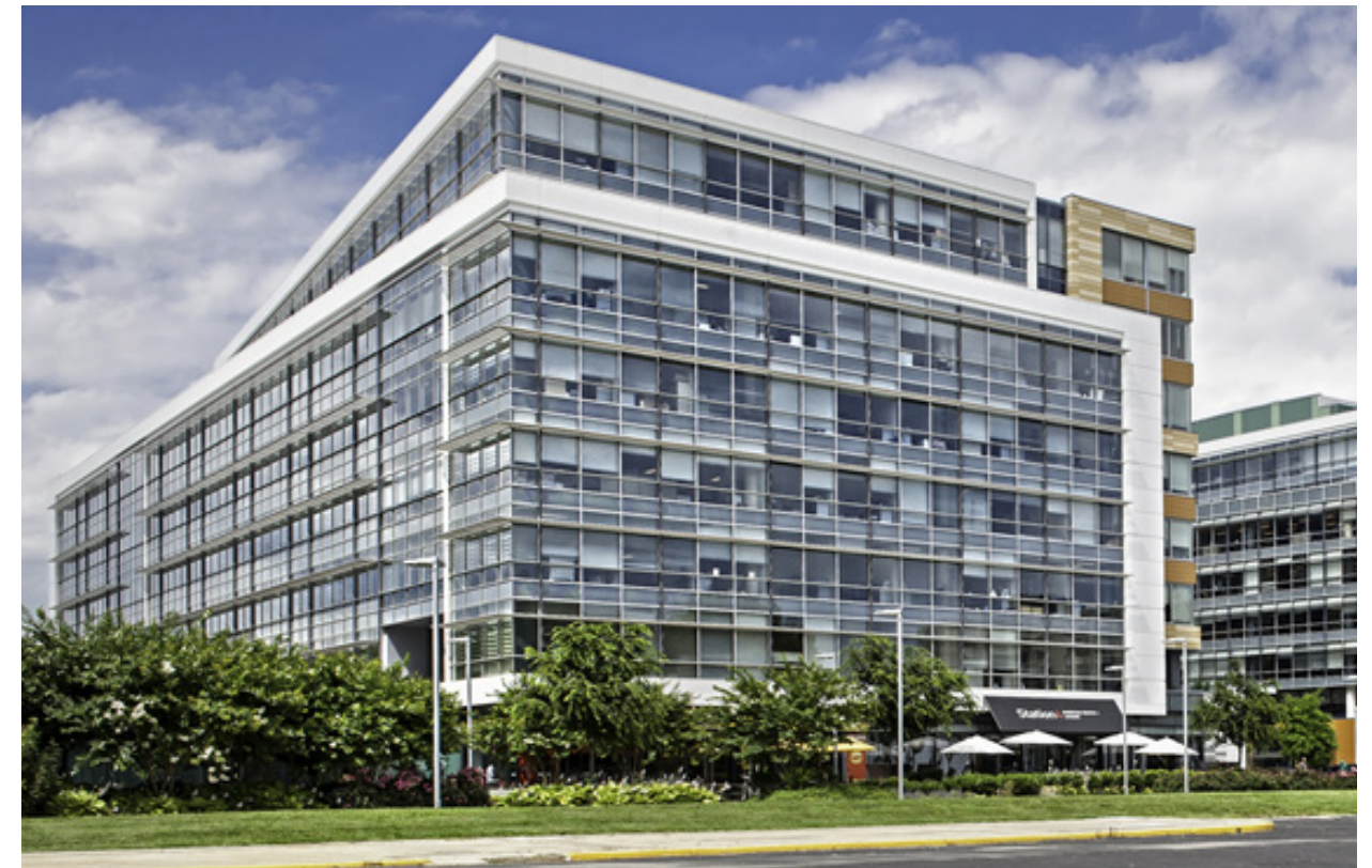
Waterfront Station (2010) - Metal Panel & Cement Panel
