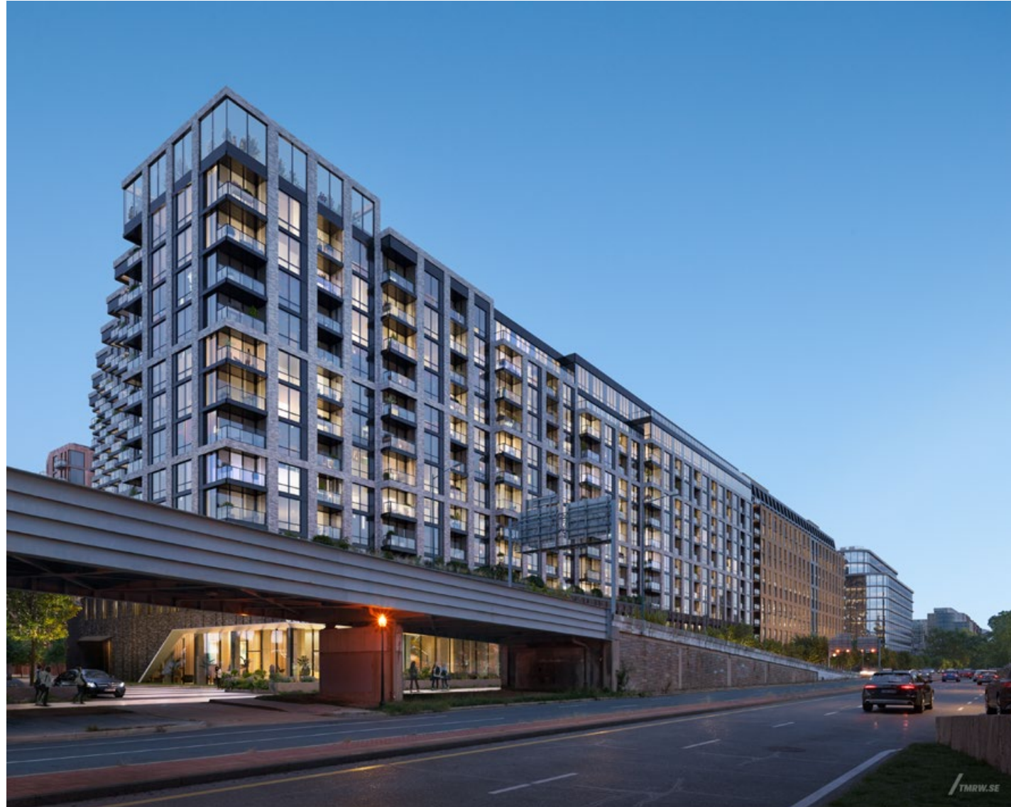
SOUTH CAPITOL ST LOOKING SOUTH - WITH RAMP
