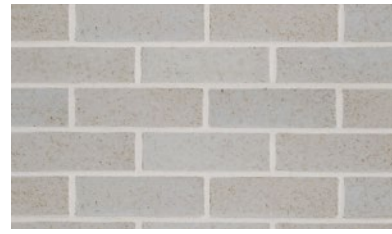
2. BRICK AT TOWER
