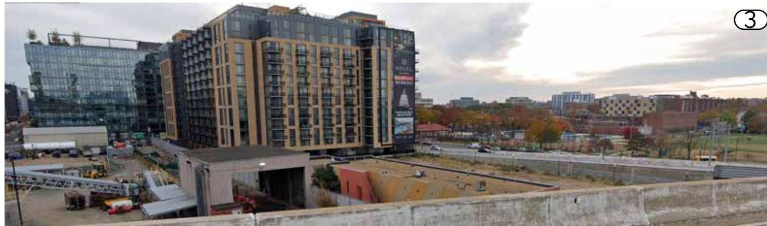
I-695 FREEWAY LOOKING SOUTH
