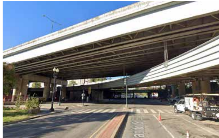
IMAGE A - EXISTING INTERSECTION NORTH OF SITE
