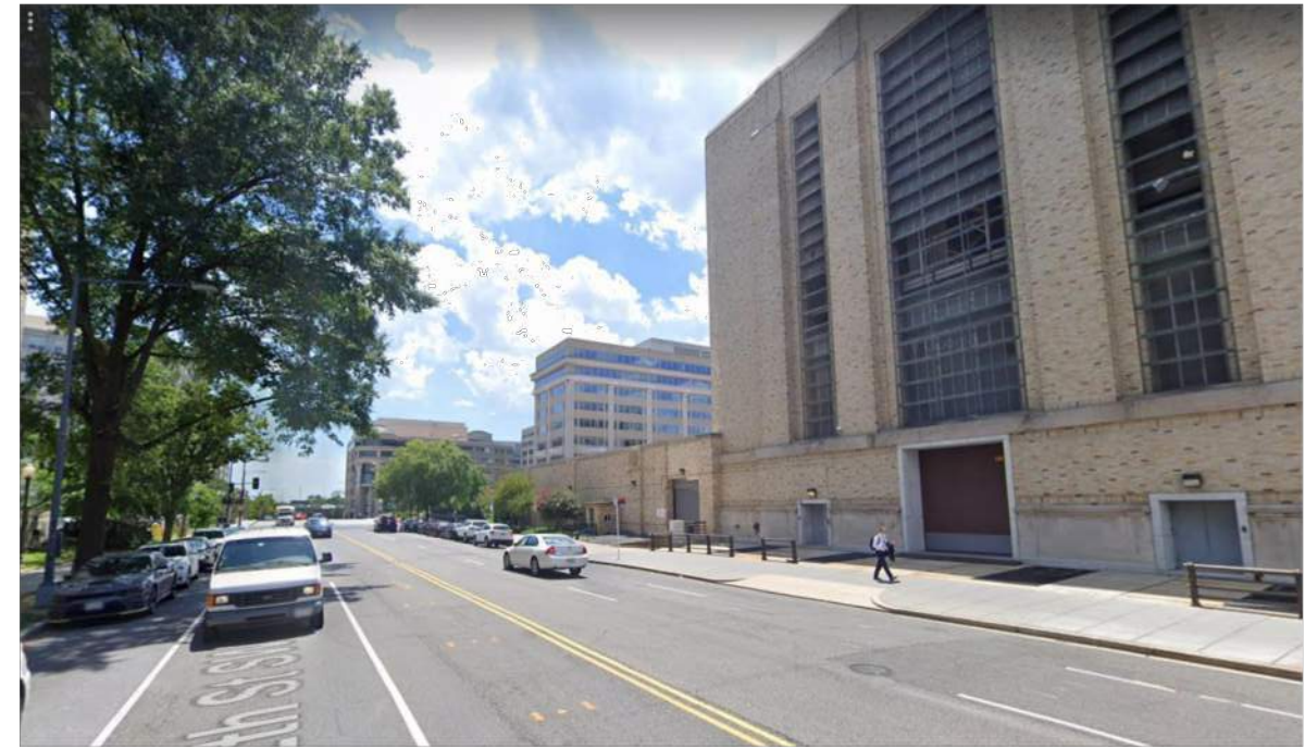
12 Street view South
