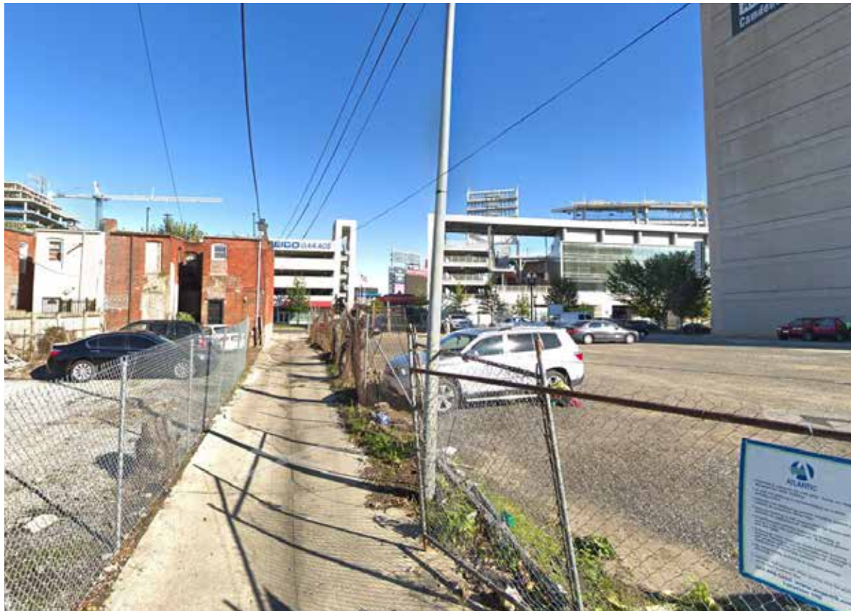
2. E/W ALLEY LOOKING EAST
