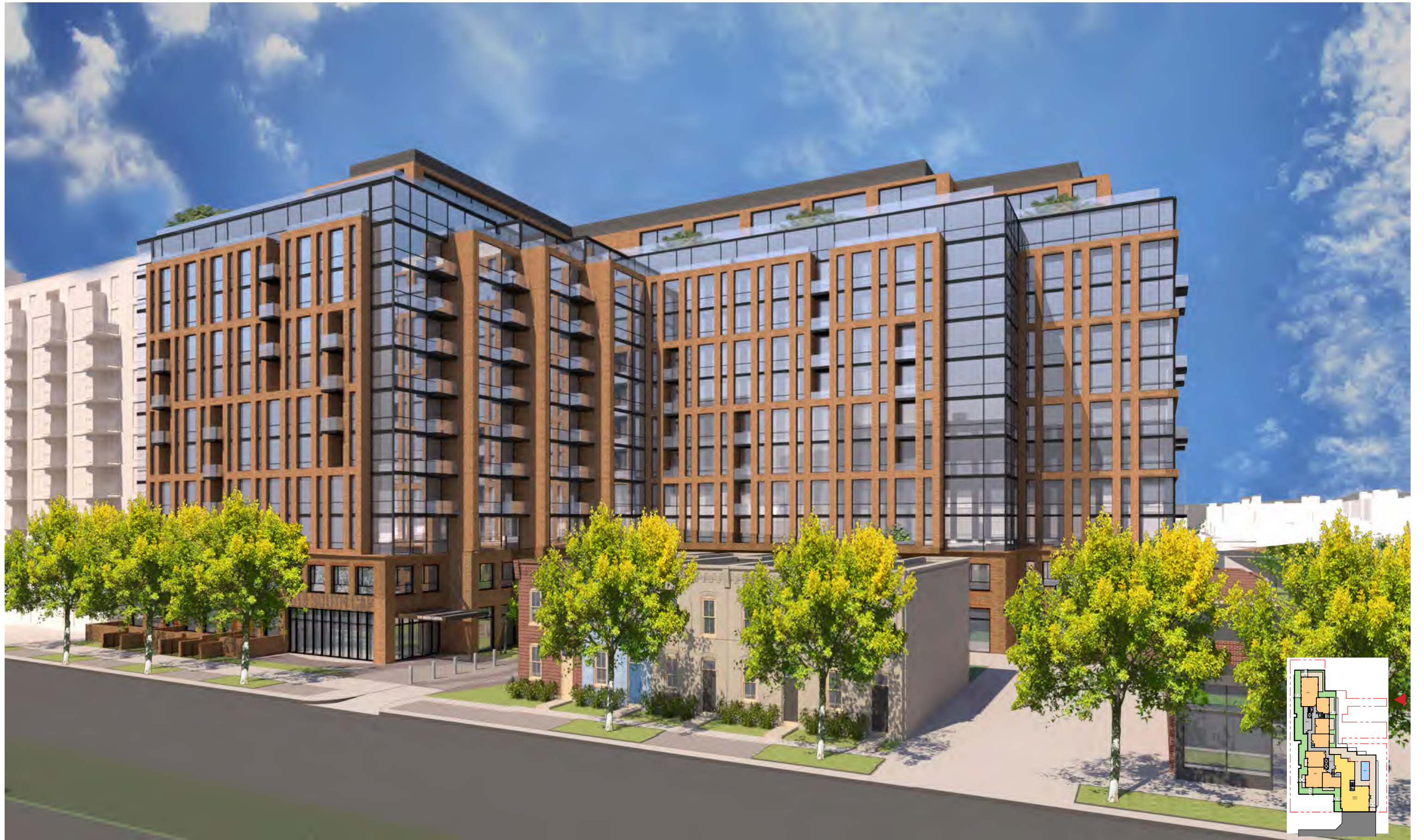
SOME PROPOSED STREET TREES HAVE BEEN REMOVED FOR ILLUSTRATION. SEE PAGE 32 FOR GLASS BALCONY DETAIL.
