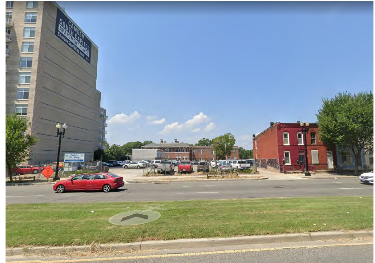
4. CURRENT PARKING LOT
