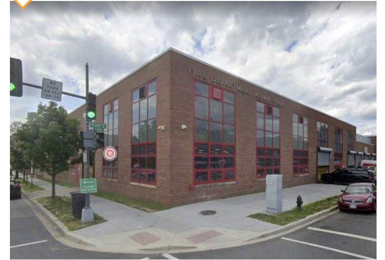
C DC Fire & EMS Station
