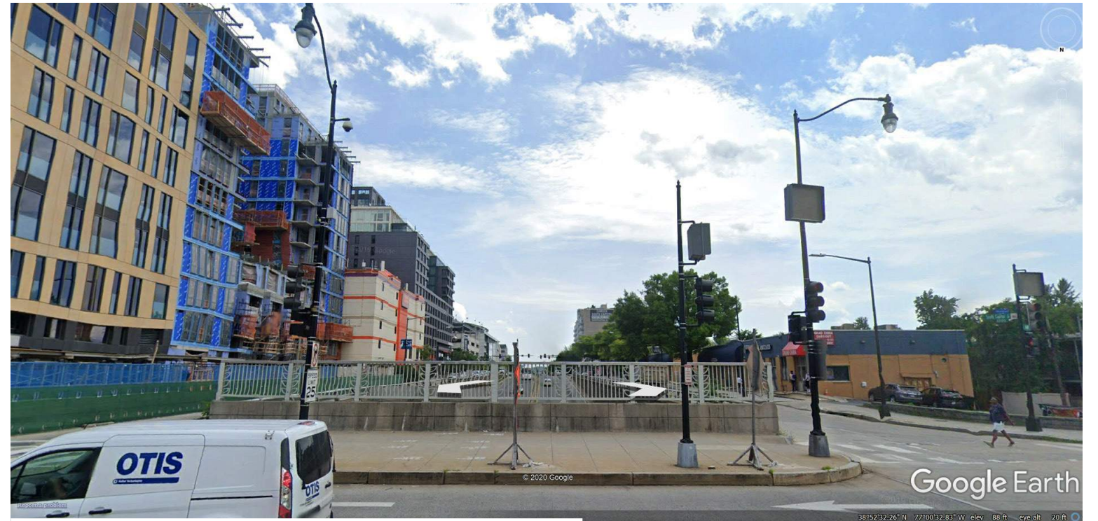
LOOKING SOUTH TO BRIDGE
