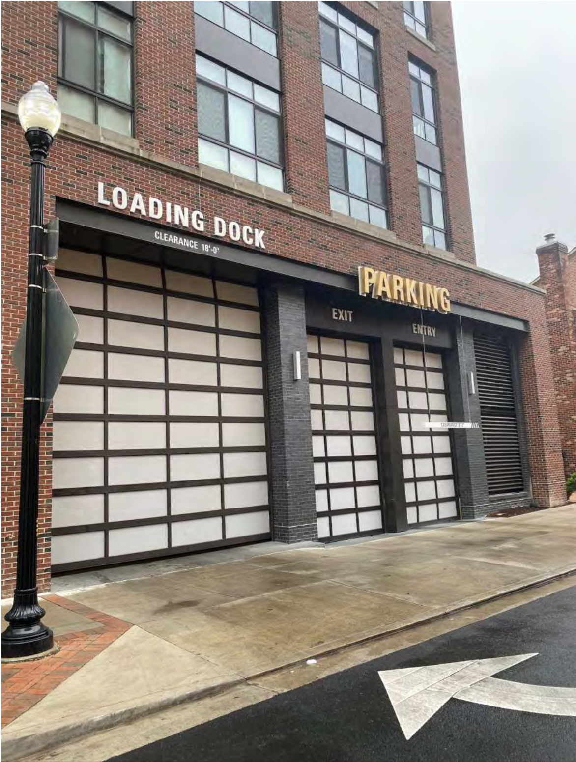
EXAMPLE OF LOADING DOCK MATERIAL
