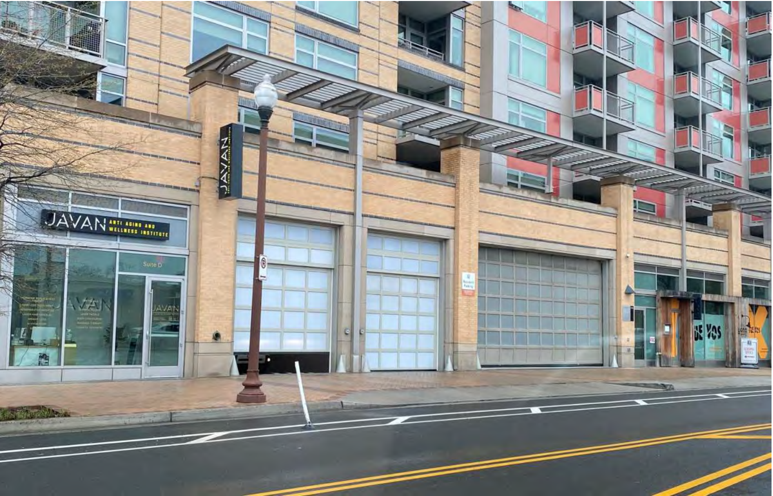
EXAMPLE OF LOADING DOCK MATERIAL
