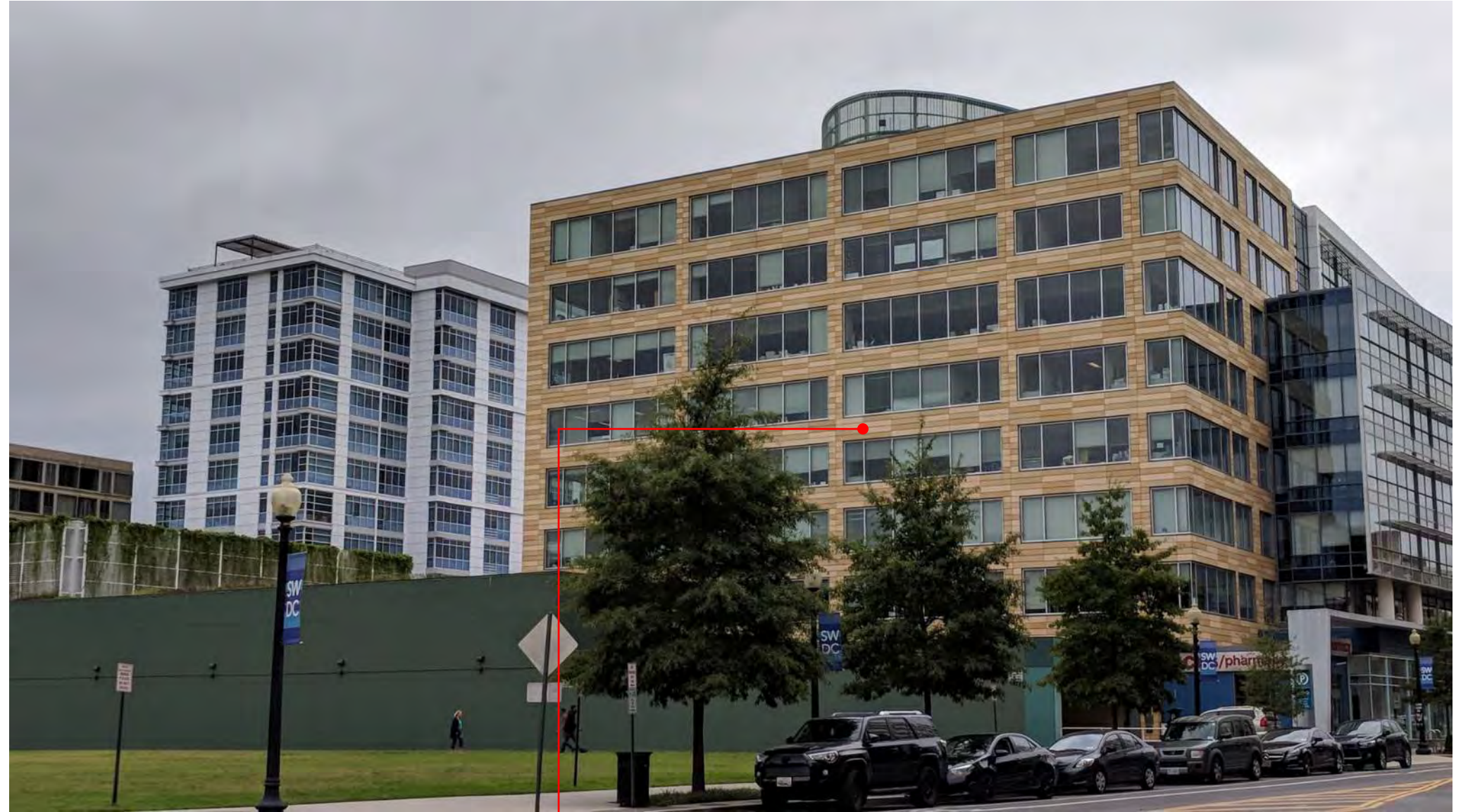
DCRA BUILDING 4TH STREET
