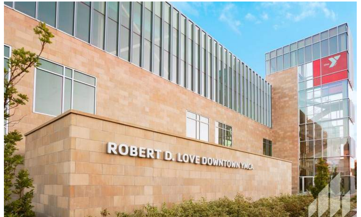
PROPOSED PREFINISHED CMU ARRISCRAFT RENAISSANCE CMU; LARGE FORMAT SIZE: 12" X 24" COLOR: SANDRIFT
