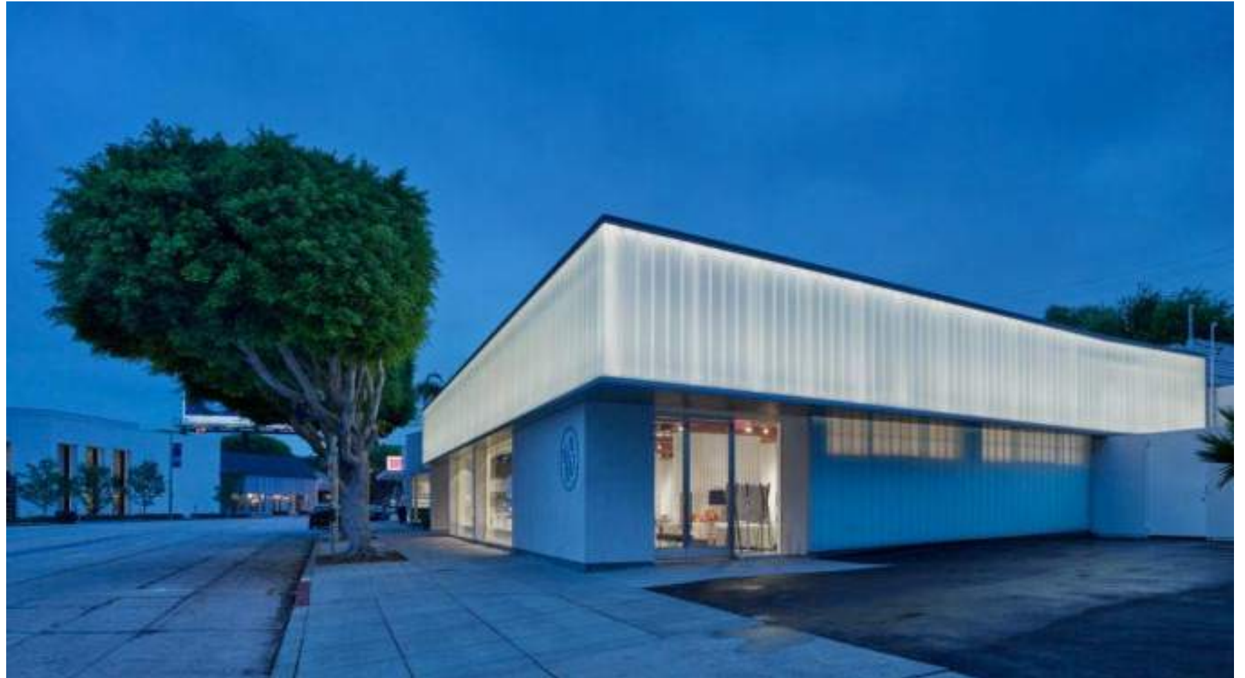
EXAMPLE CONTINOUS BACKLIT CHANNEL GLASS MATERIAL (FC LEVEL OF LIGHTING IS UNKNOWN)
