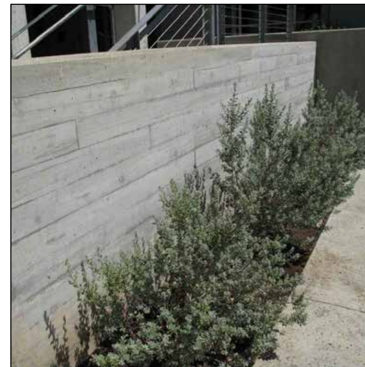
BOARD FORM CONCRETE RETAINING WALL
