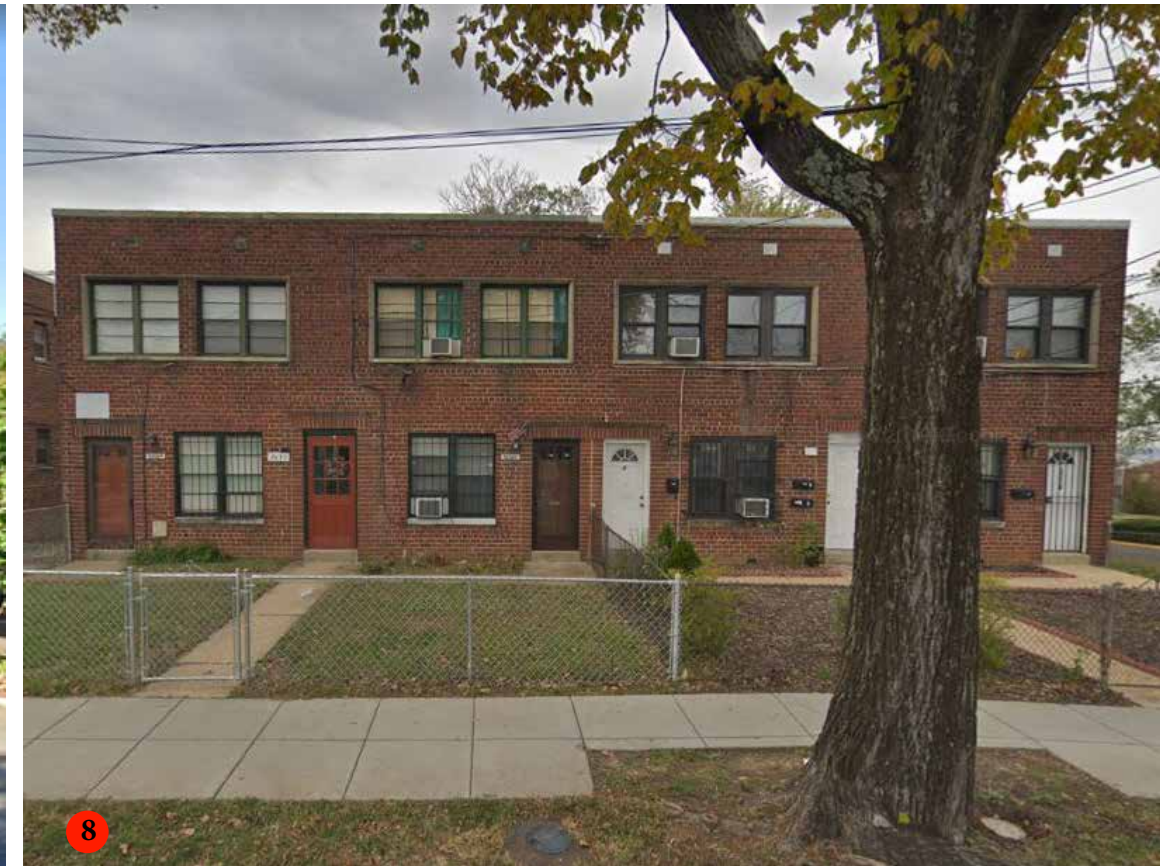
View south down 25th st SE of adjacent homes
