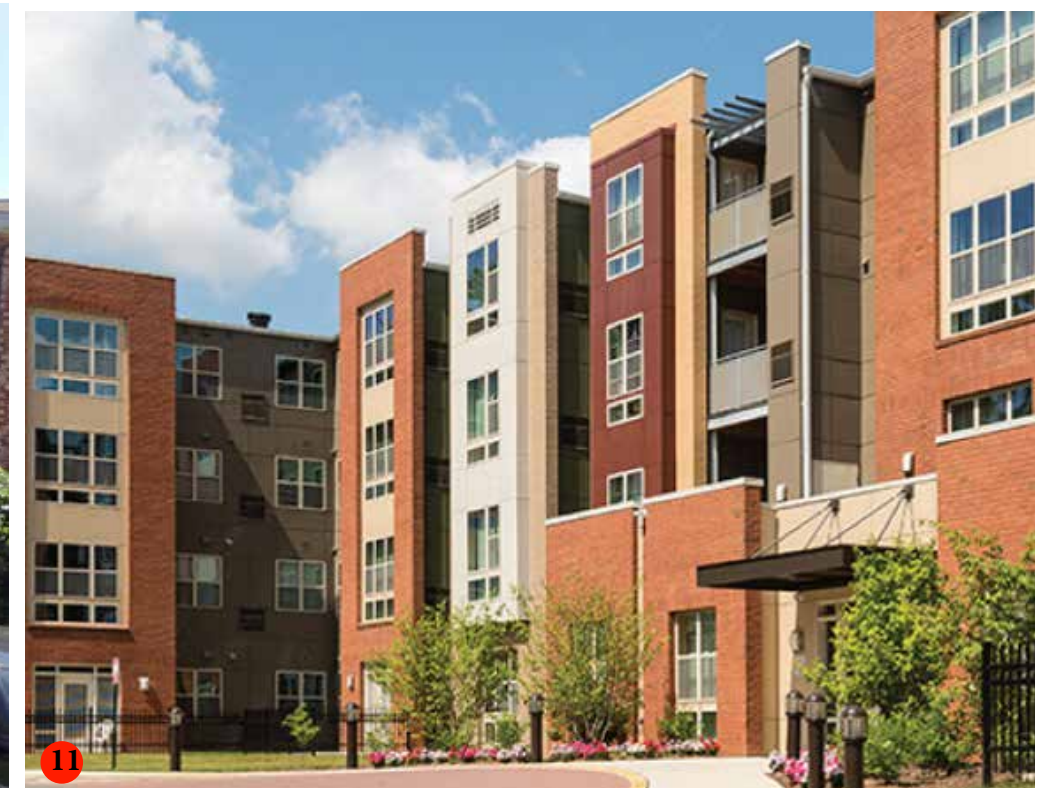
View North up Alabama Ave SE - Roundtree Residences
