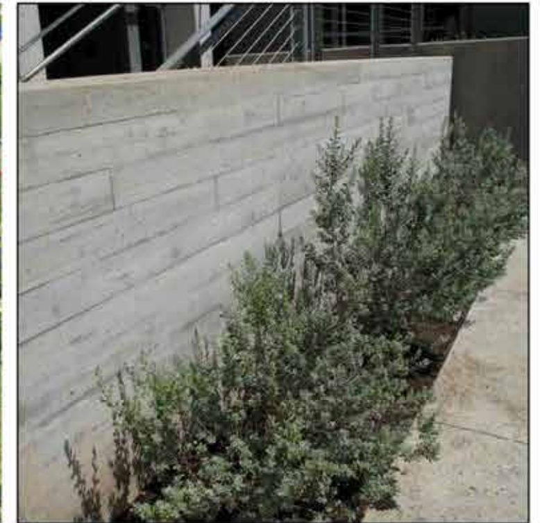
BOARD FORM CONCRETE RETAINING WALL
