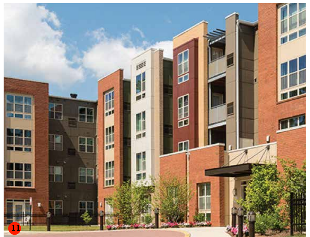
View North up Alabama Ave SE - Roundtree Residences
