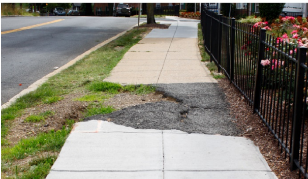
E | Cracked pedestrian pathway along 25th Street south of Good Hope Road SE
