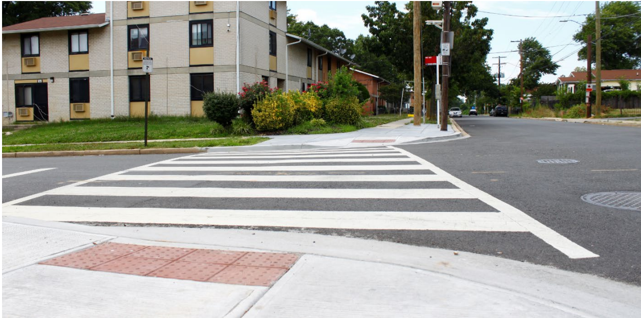
Figure 9: Curb Ramps at Good Hope Road SE and 24 th Street SE lack Truncated Domes
