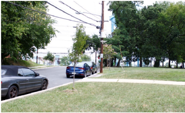
A | Sidewalk not provided on south side of Wagner Street SE
