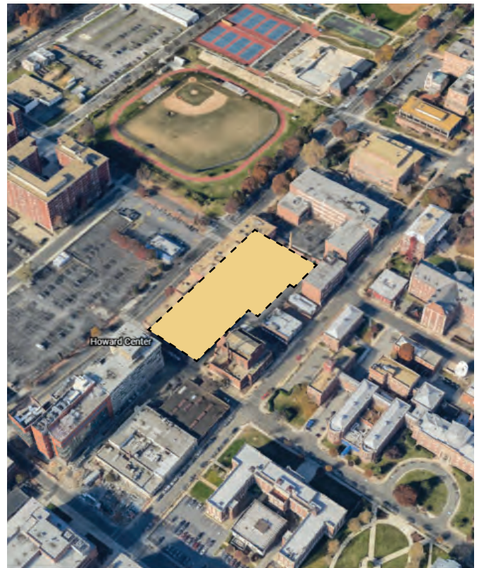
Figure 4.34: Fusion Building in Context
