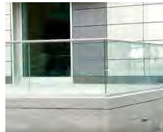
5. ROOFTOP GLASS RAILINGS
