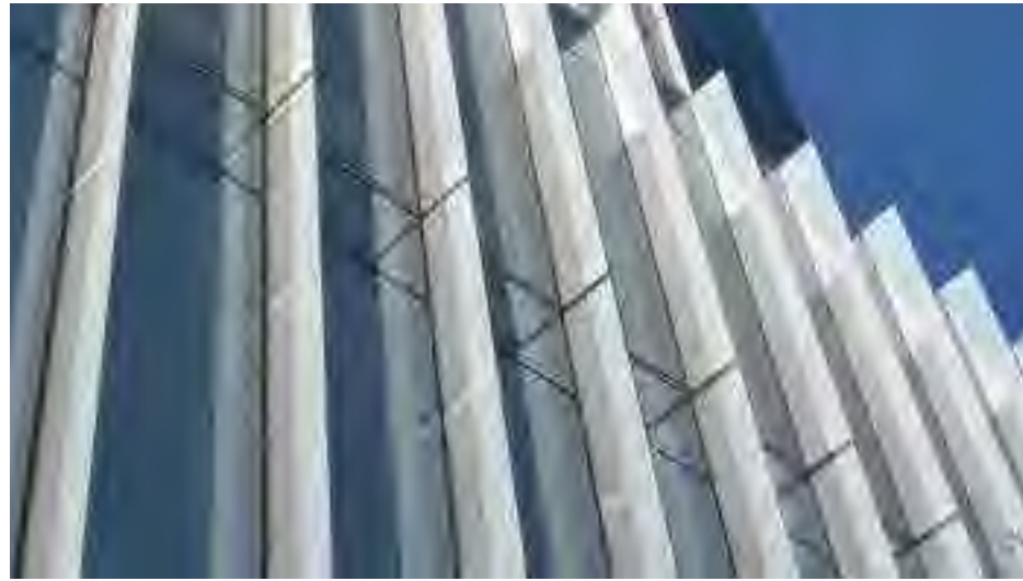
6. FIN EXTENSIONS AT CURTAIN WALL
