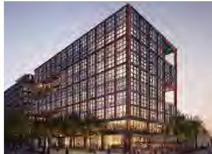
Signal House - Carr
