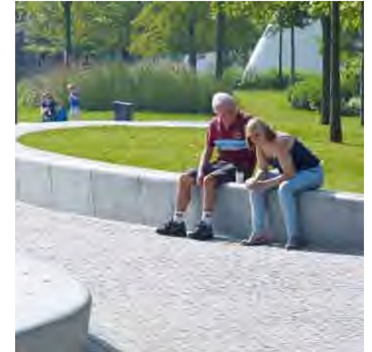
C.I.P. CONCRETE SEATWALL
