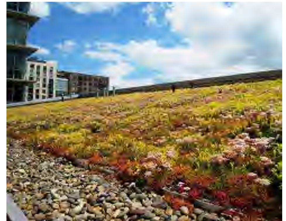
SEDUM PLANTING AT NON-ACCESSIBLE ROOF SPACES
