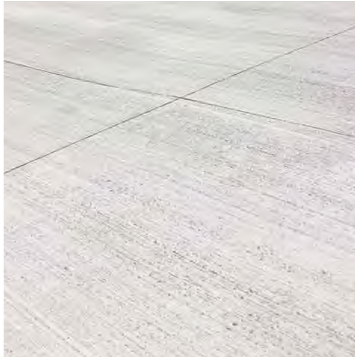
STANDARD BROOM FINISH CONCRETE, 5' X 8' SCORING
