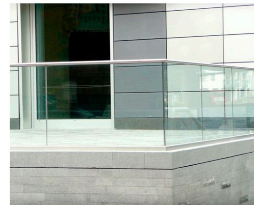
5. ROOFTOP GLASS RAILINGS
