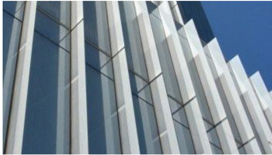
6. FIN EXTENSIONS AT CURTAIN WALL
