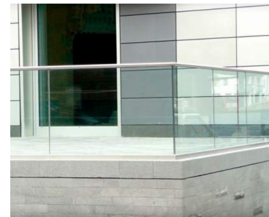
5. ROOFTOP GLASS RAILINGS
