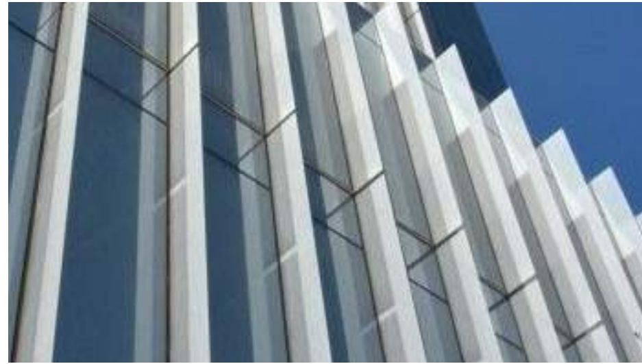
6. FIN EXTENSIONS AT CURTAIN WALL
