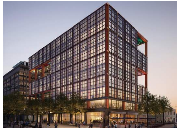
Signal House - Carr
