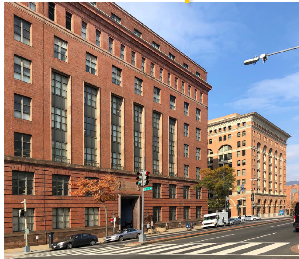
Government Printing Building (South of Site)
