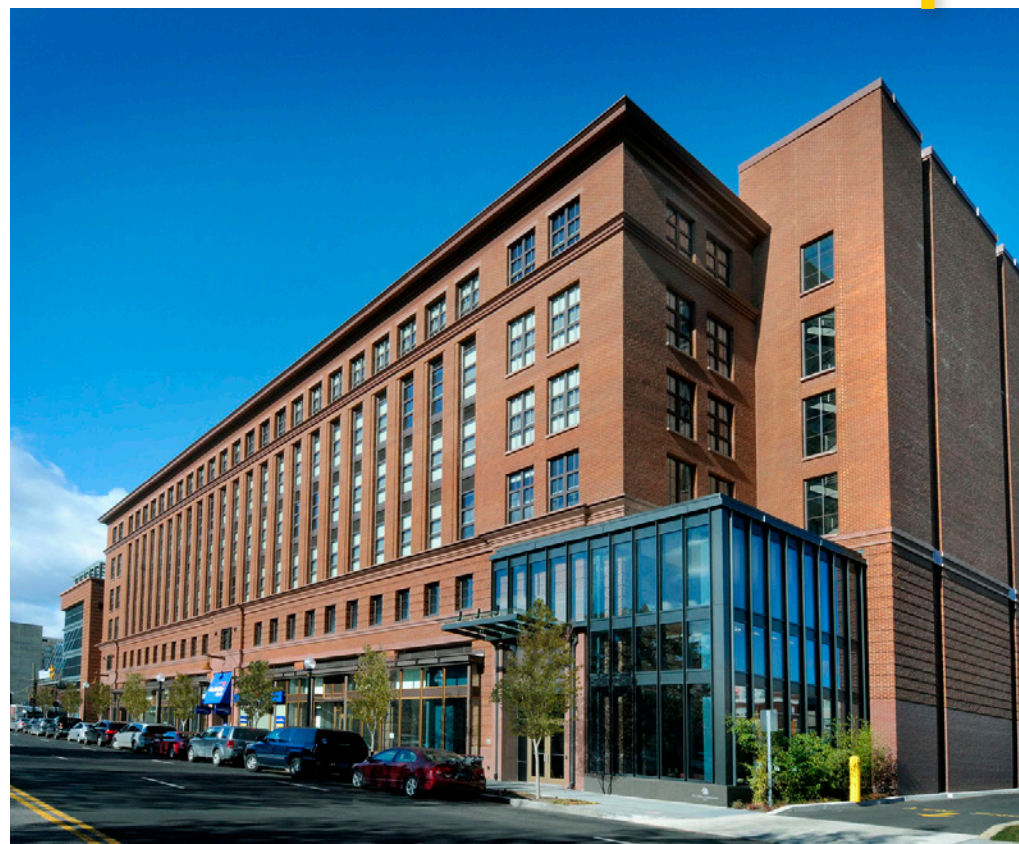
77 H Street (West of Site)
