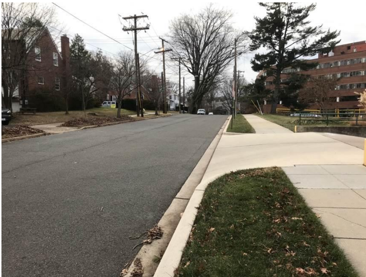
The next photo shows the ramp and the retaining wall that holds up the 48th Street embankment:
