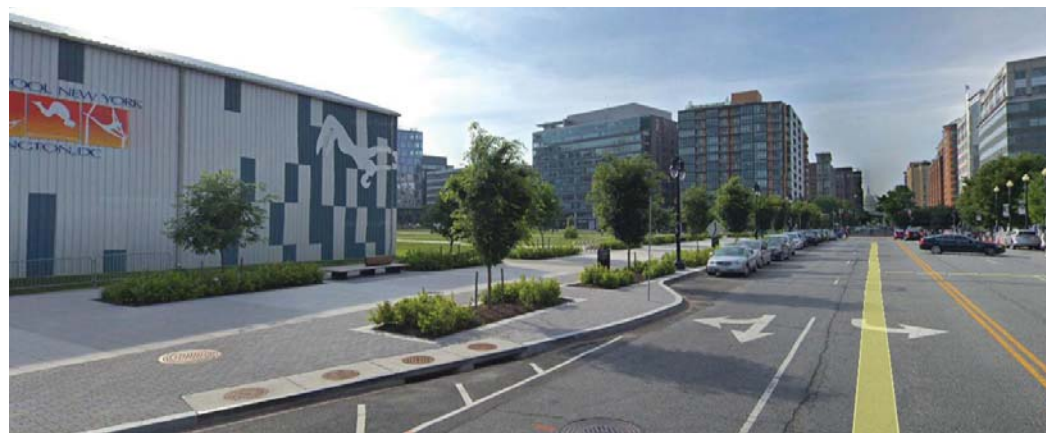
Concrete Pavers on New Jersey Ave
