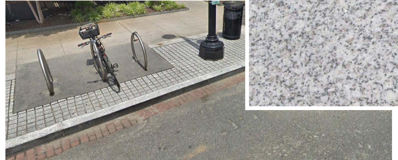
Mount Airy Granite Curb and Cobble standard to the Yards and DC
