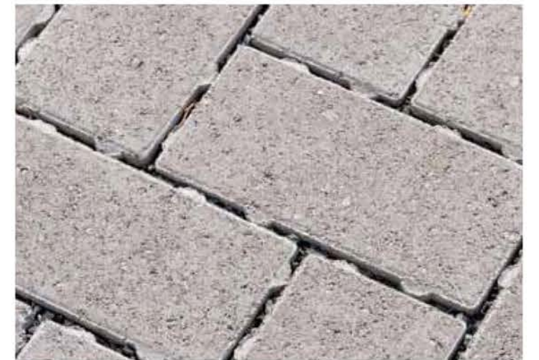
PERMEABLE PAVING
