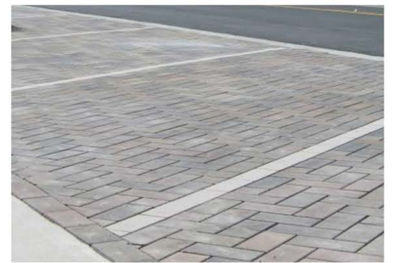
PERMEABLE PAVING
