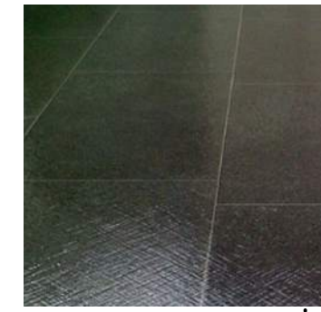
BLACK GRANITE PAVING
