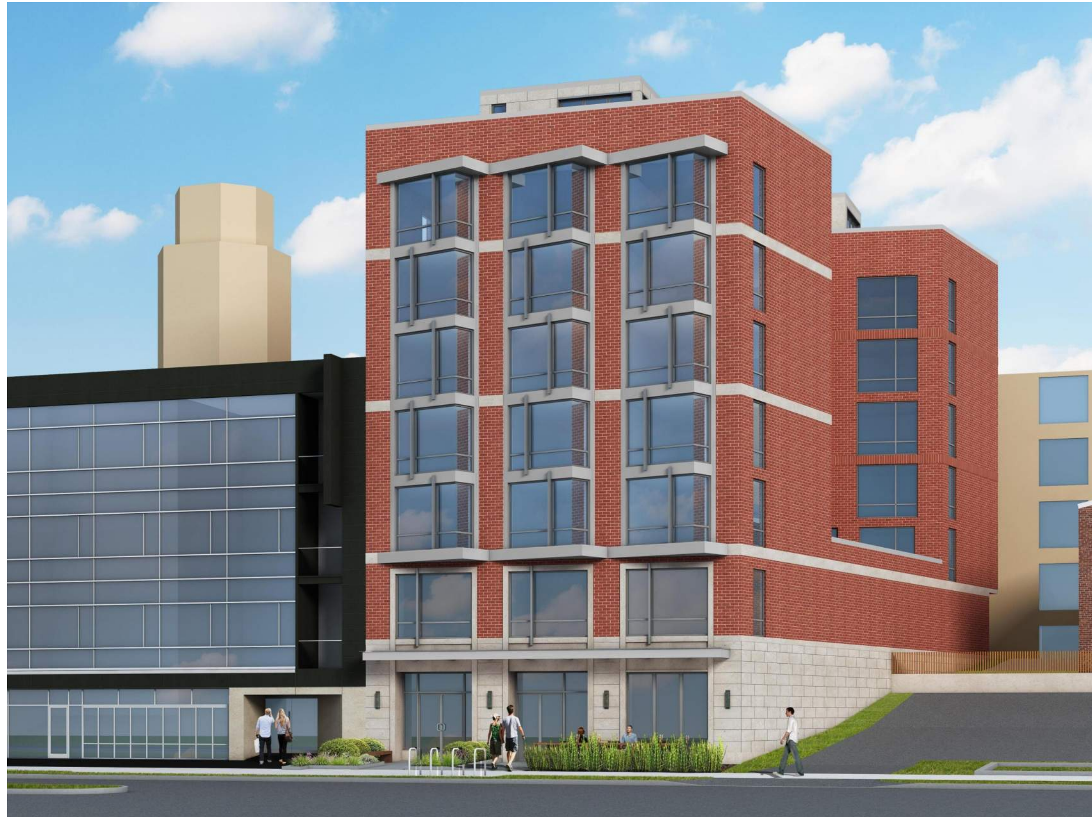
VIEW LOOKING NORTHEAST
