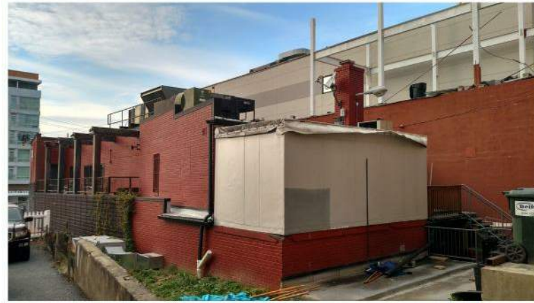
4. View from alley looking northwest
