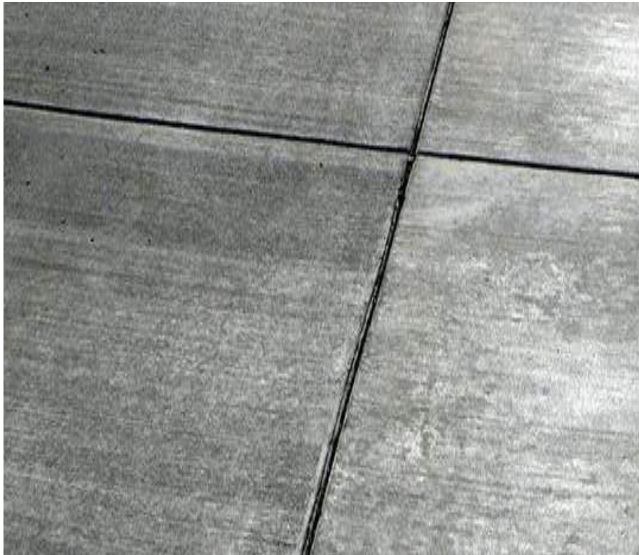
CONCRETE SIDEWALK: 5'x8' Scoring, Hairbroom Finish
