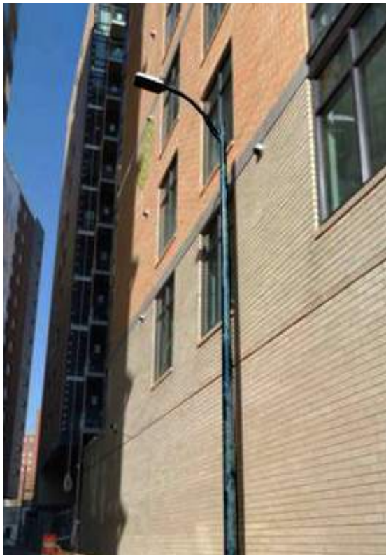
STREET LIGHT: COBRA HEAD - PHILIPS/VALMONT - ROADVIEW LED
