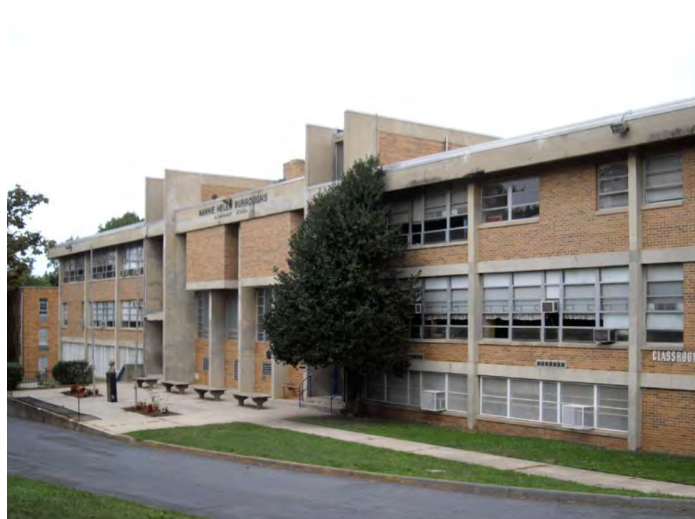
H School Building
