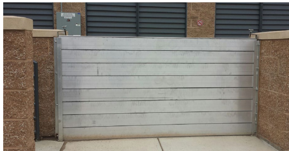
1. Typical Flood Plank, FP-530 by PS Doors
