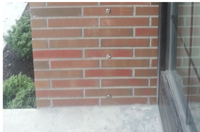
2. Pre-bolted connection for a completely removable system
