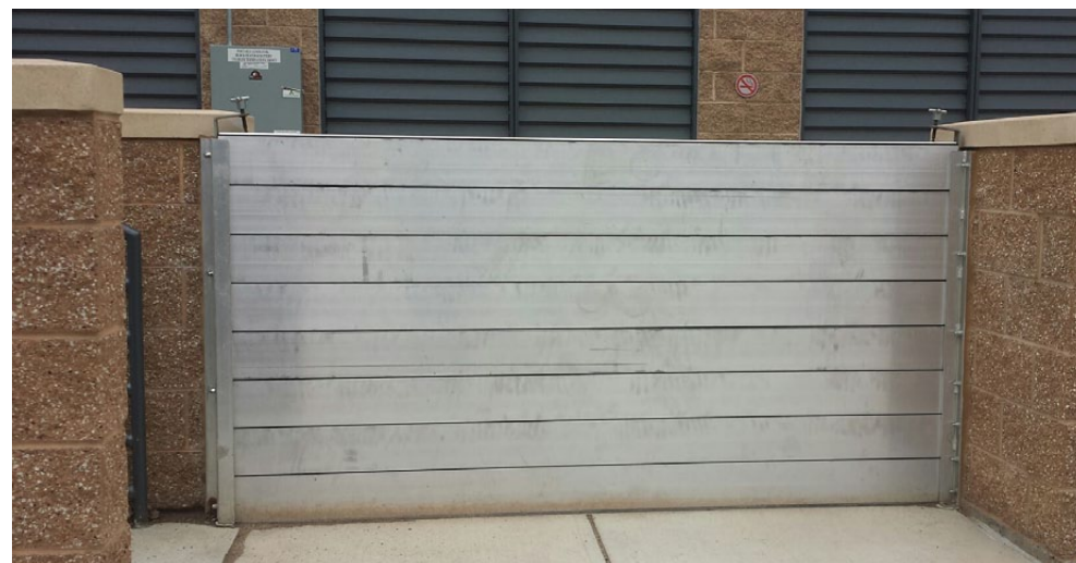
1. Typical Flood Plank, FP-530 by PS Doors
