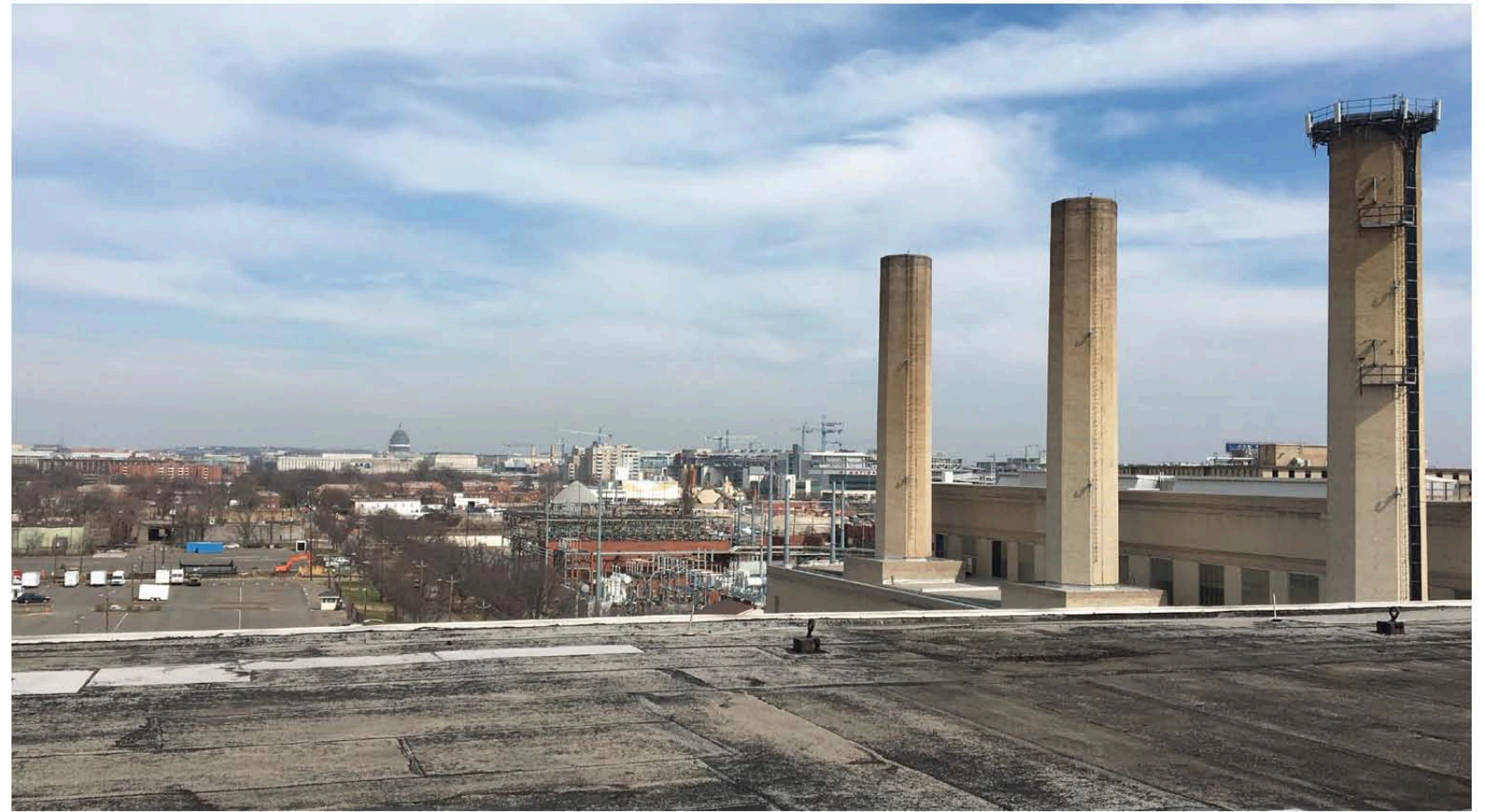
2. VIEW FROM NORTHEAST CORNER
