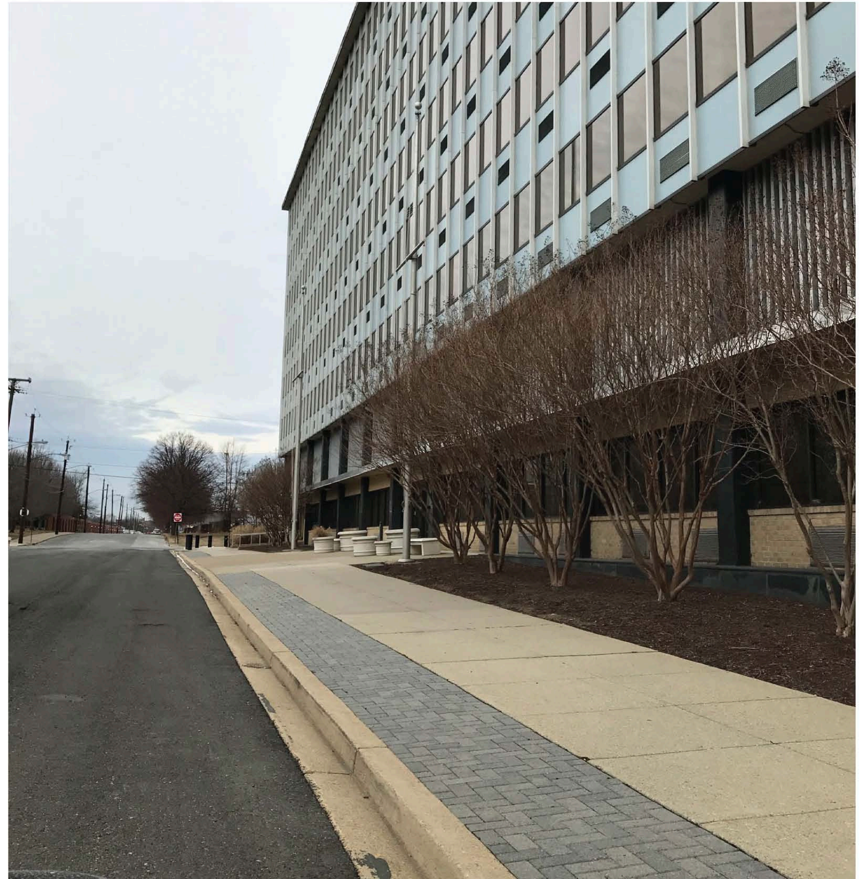
4. LOOKING NORTH ON 2ND ST, SW
