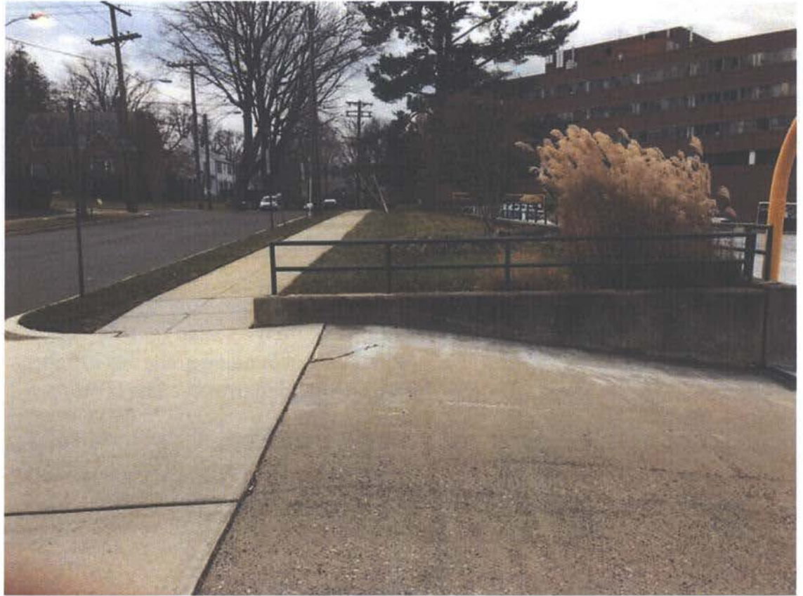
48 th Street Embankment
