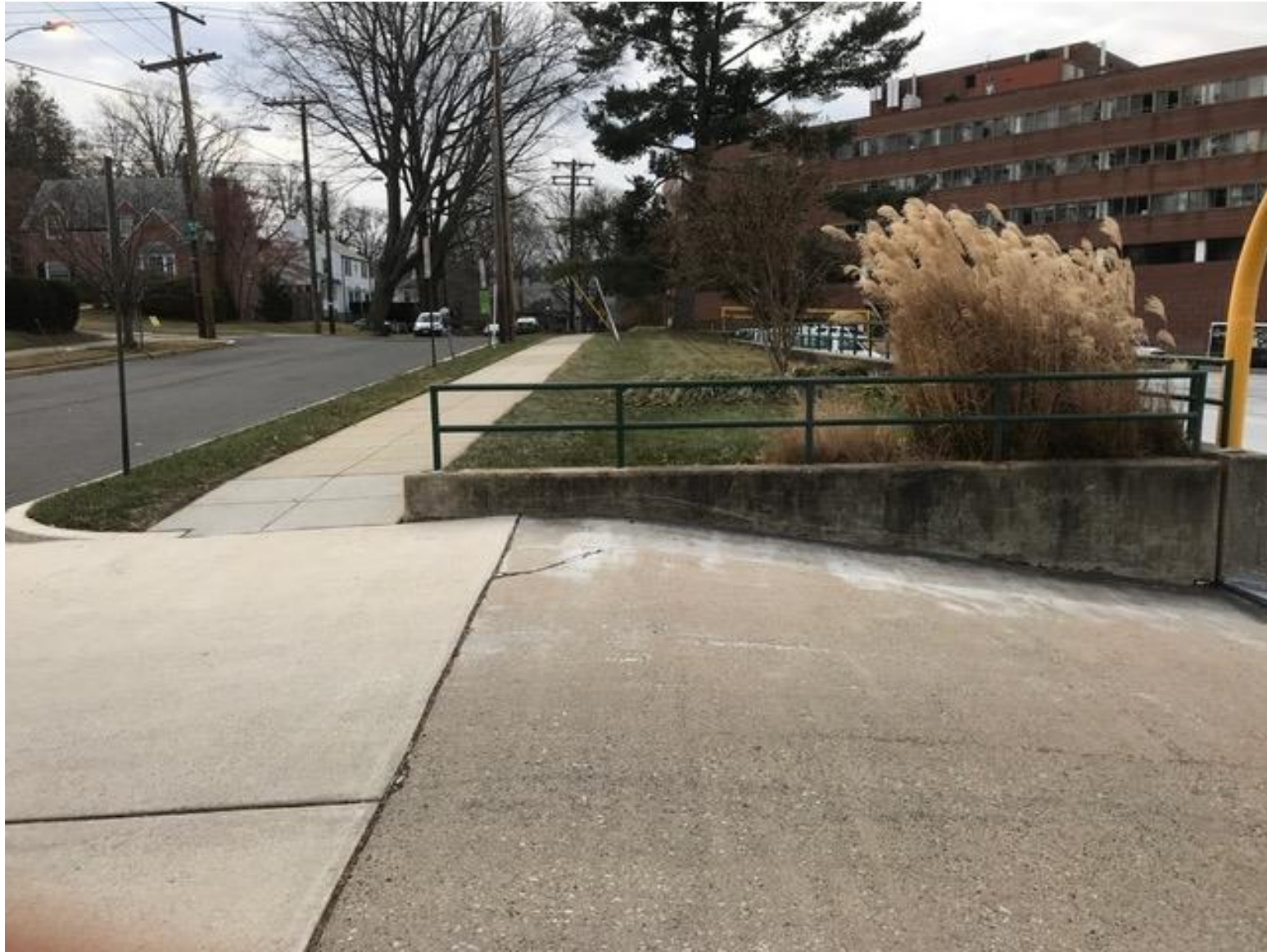
48 th Street Embankment
