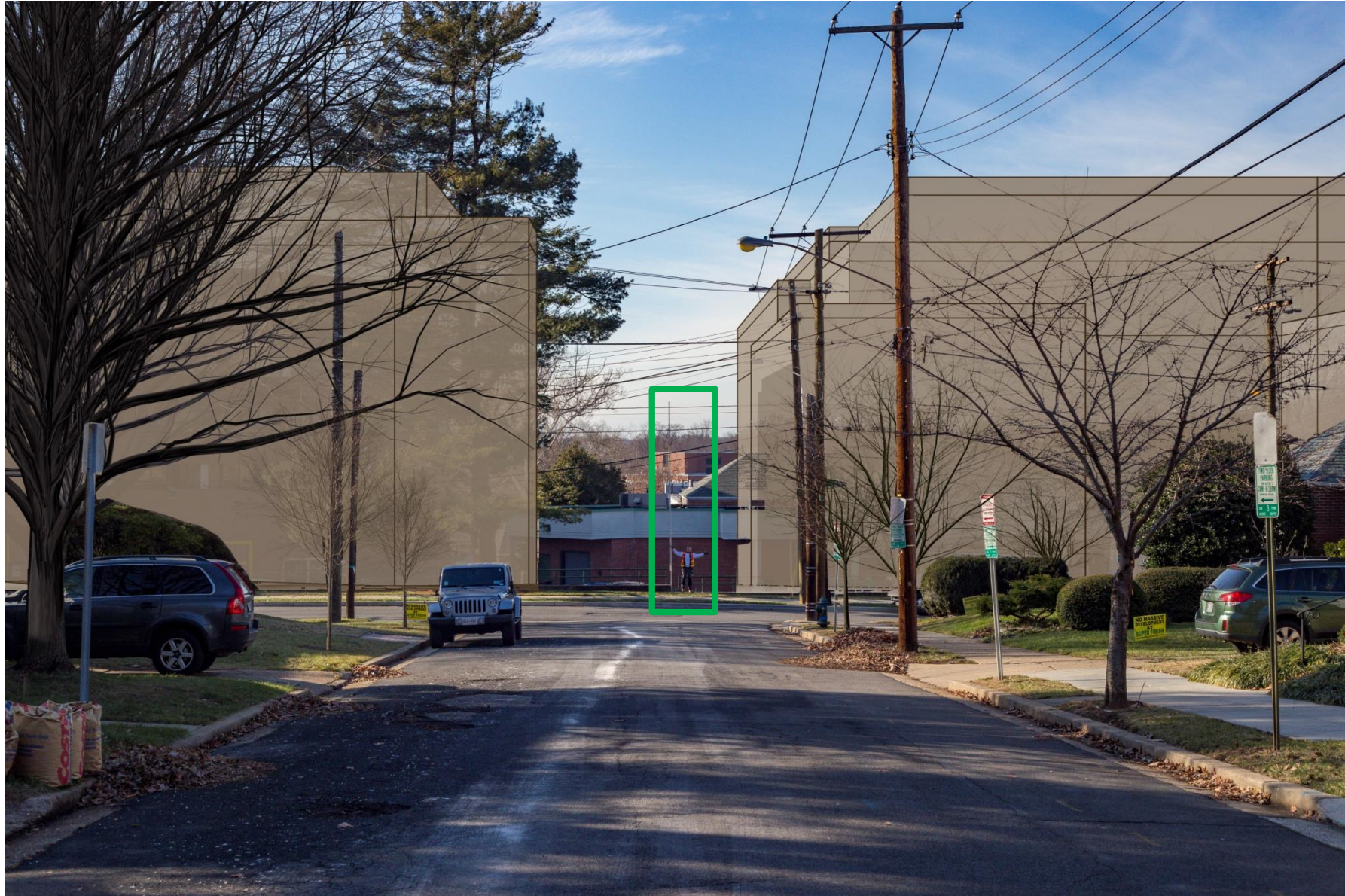
12-21-2017 Design as seen from Camera Loc. 01. The 3D model's massing accurately represents the height and width of the proposed development from this Windom Pl perspective. A 25ft tall survey rod is held by surveyor.
