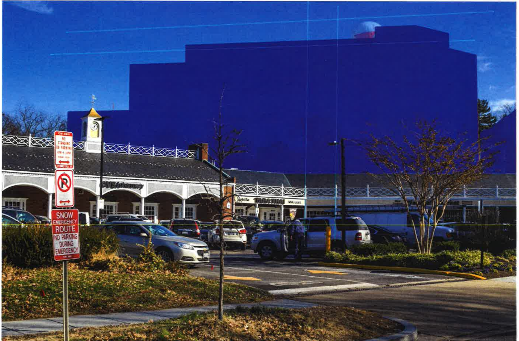
The blue transparent 3D massing model represents the Ladybird's height and width relative to the historic shopping center.
