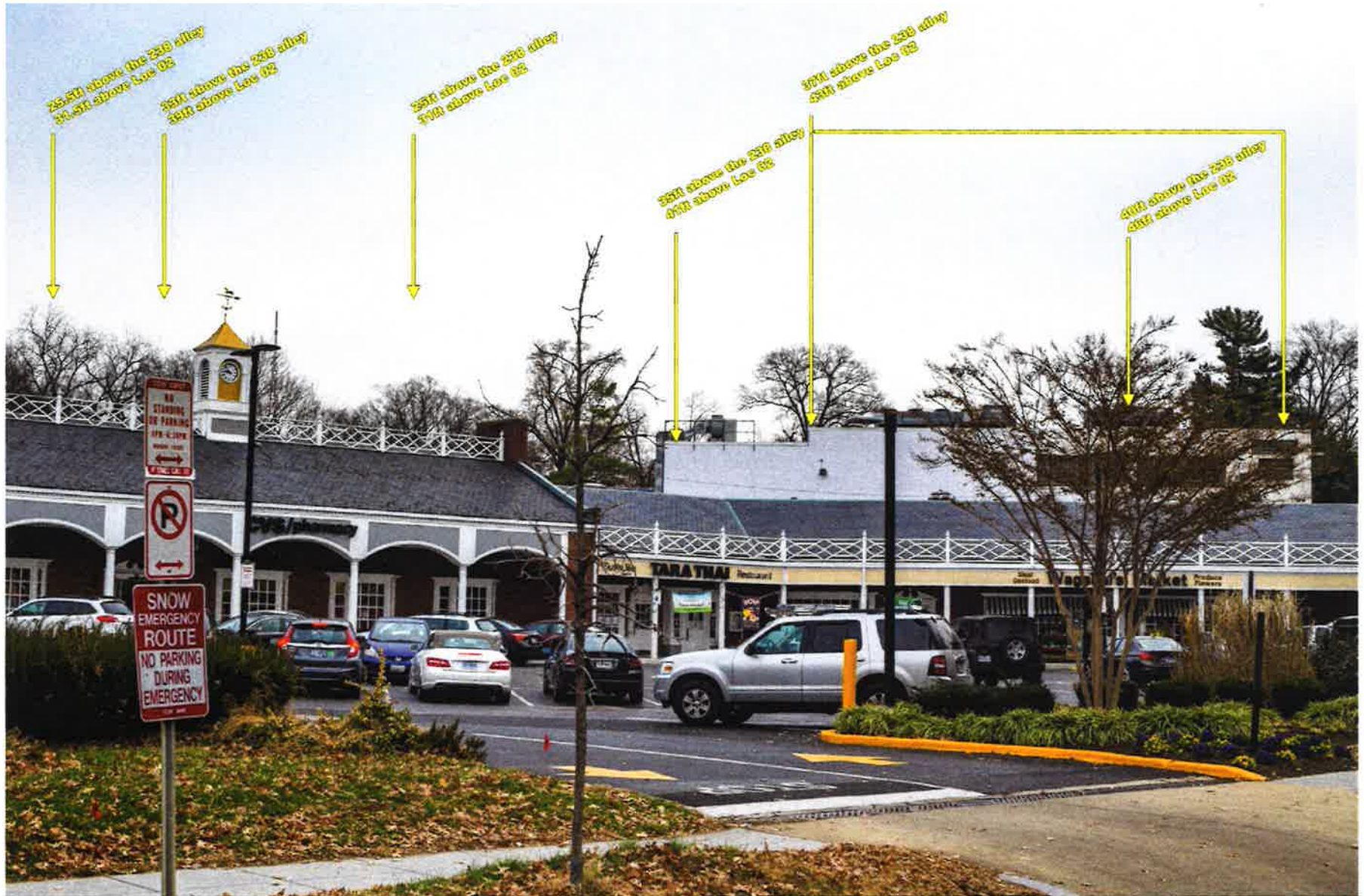
Laser Measurements of the existing structures (in yellow) were taken to use as references when verifying the 3D Model's placement and scale.
