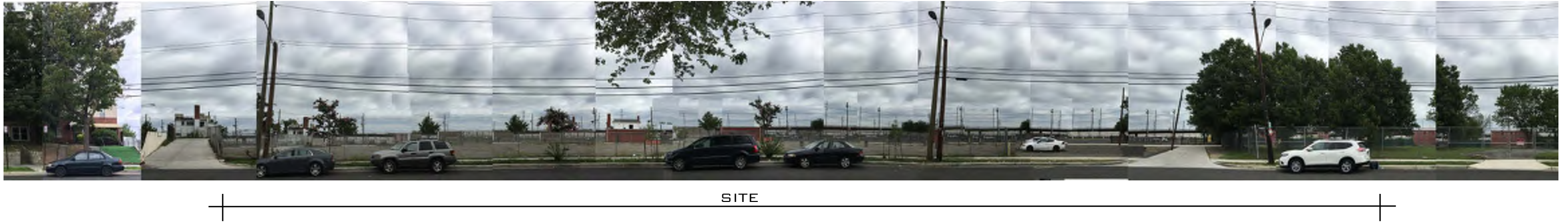
1 | EADS STREET ELEVATION LOOKING NORTH
