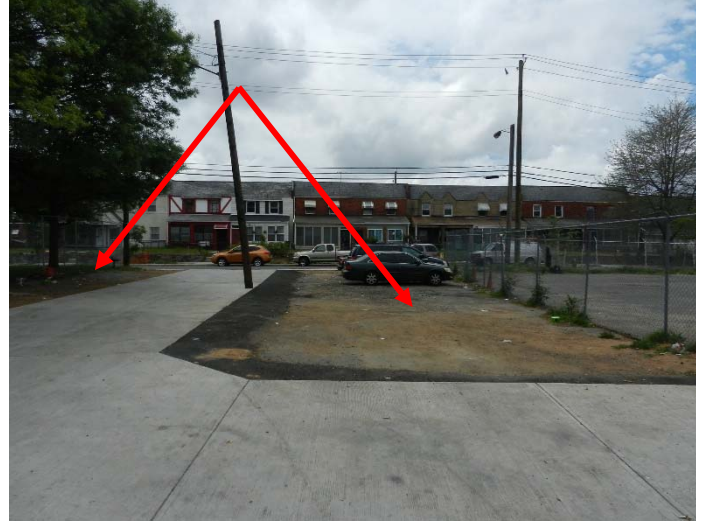
8. View of the two non-paved and unfenced portions of the Property located along Eads Street
