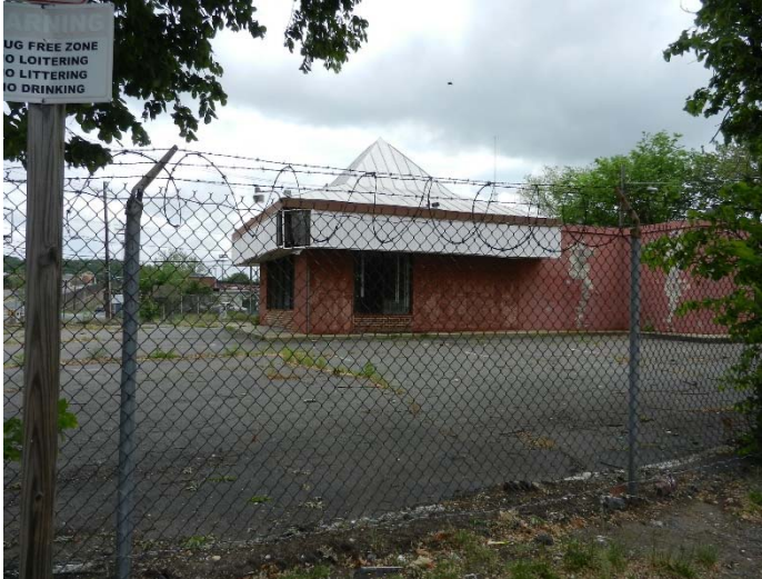
5. View of the adjacent former gas station and auto repair facility to the northeast
