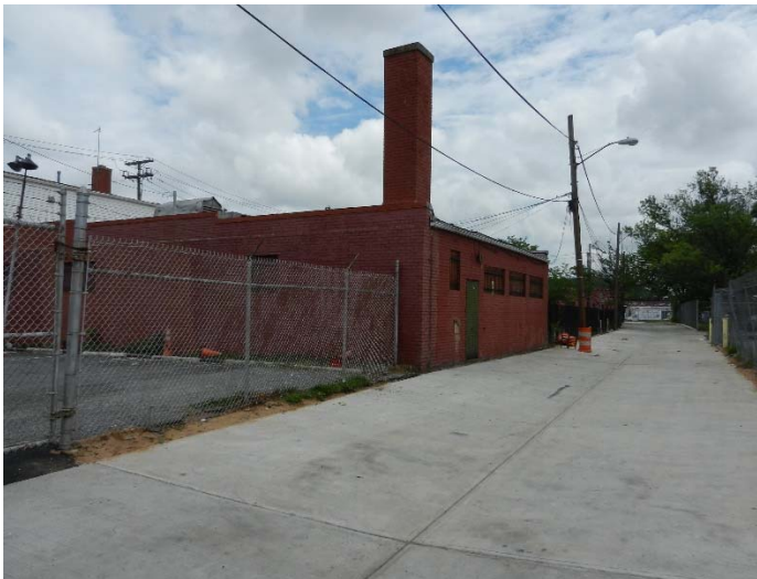
13. View of the rear of Benning Liquors looking east along the alley between the northern and southern portions of the Property
