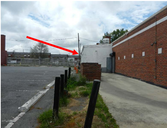
1. View of the small concrete block structure located on the western side of the northern fenced lot
