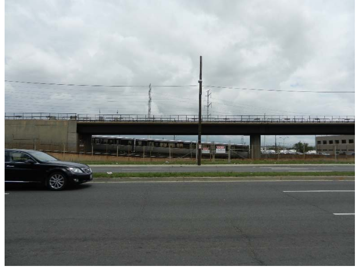
12. View looking north across Benning Road to the Metro tracks and the PEPCO generating facility
