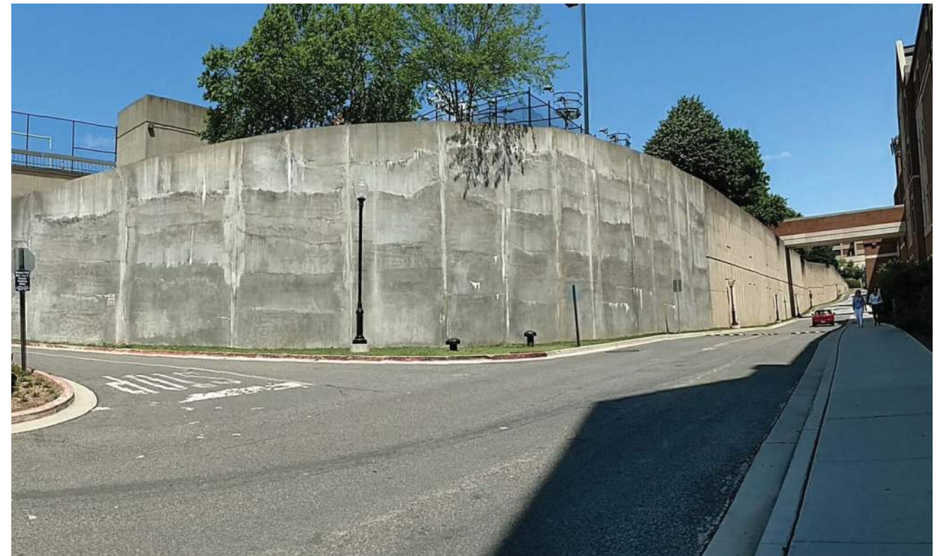
4B - VIEW LOOKING NORTHWEST
