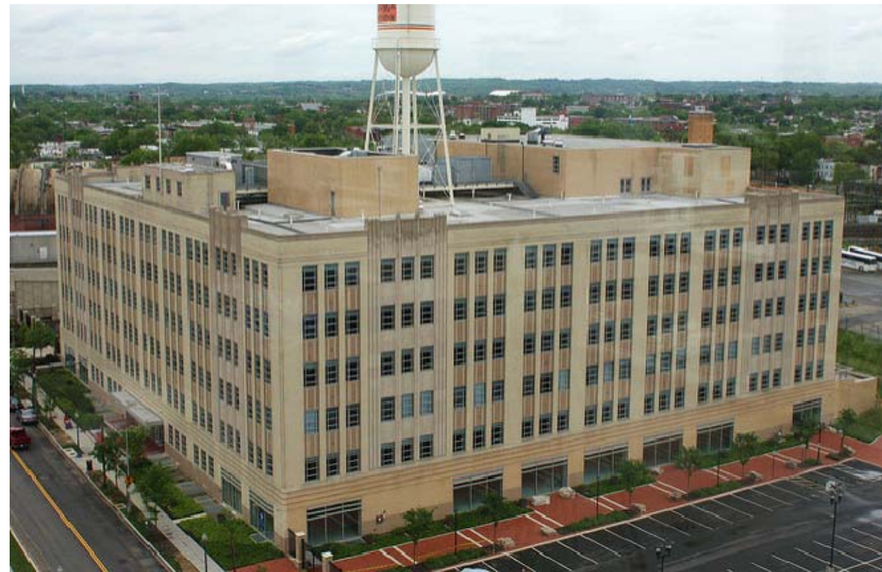
WOODWARD & LOTHROP WAREHOUSE
