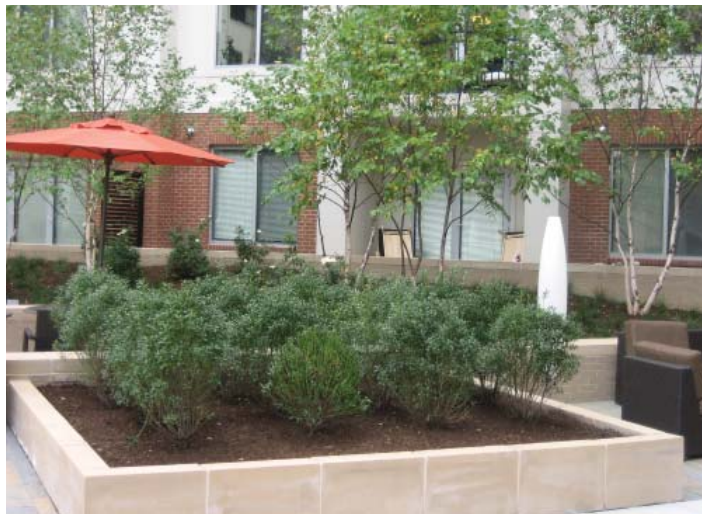
INTENSIVE GREEN ROOF WITH PLANTINGS
