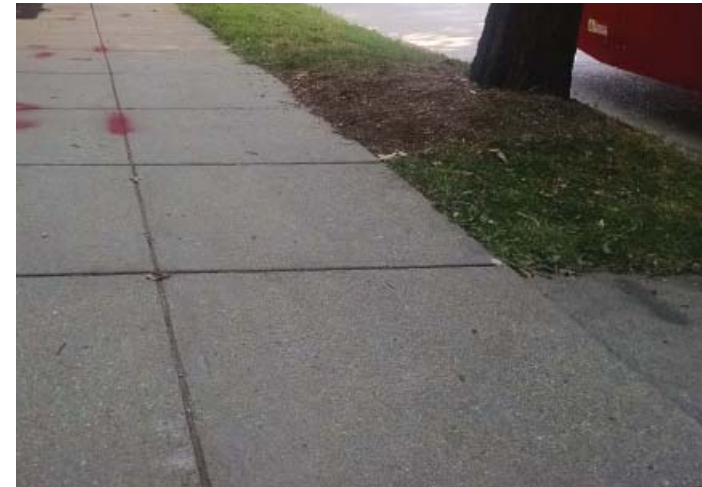
DC STANDARD CONCRETE PAVING
