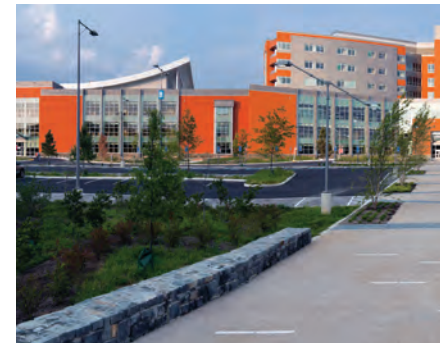
Fort Belvoir Community Hospital, Fort Belvoir, VA
