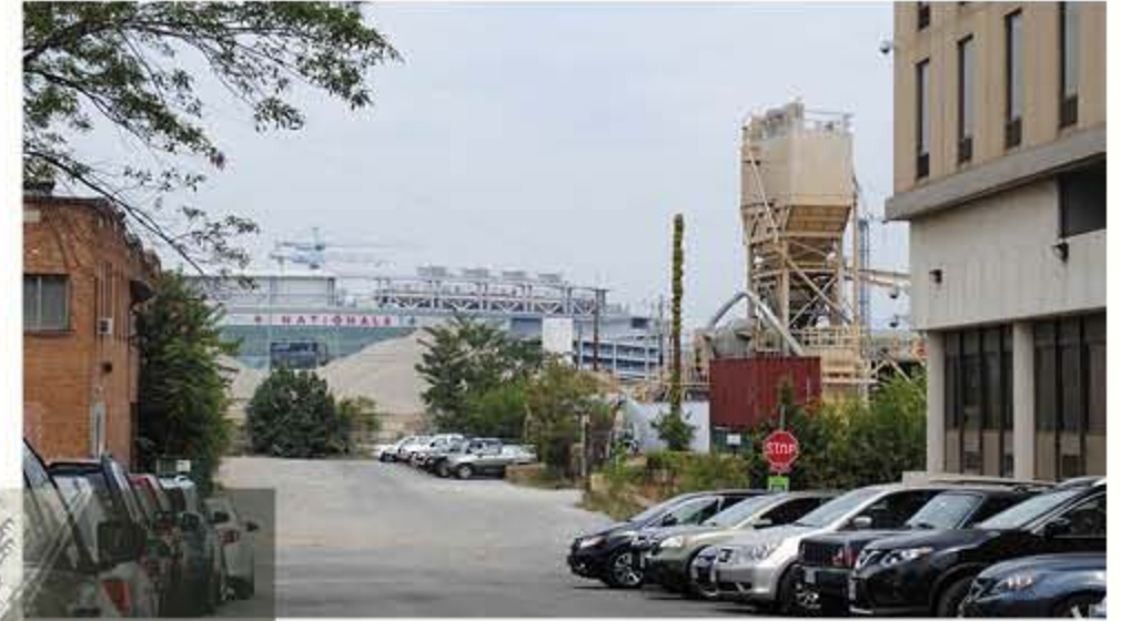
B. VIEW DOWN WATER STREET TOWARDS NATIONAL'S PARK
