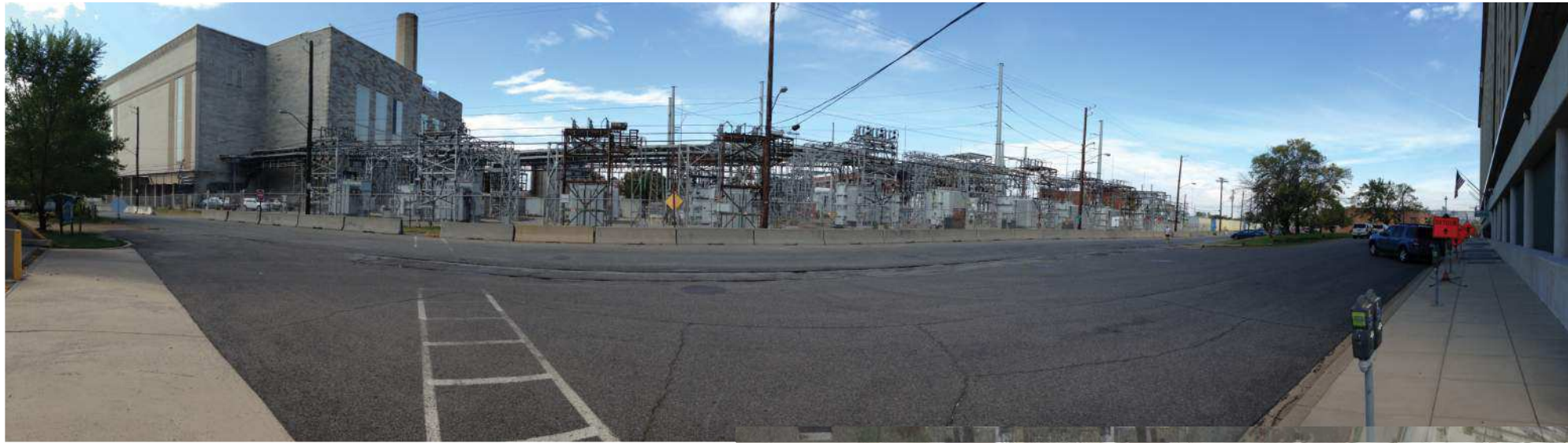
A. PANORAMIC VIEW FROM MAIN BUILDING ENTRY
