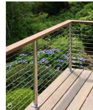
8 RAILING AT UPPER RETAIL PLAZA ALONG MASS. AVE
