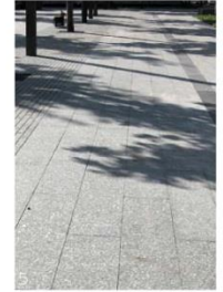
CONCRETE PAVERS AT PLAZA IN A VARIETY OF SIZES AND COLORS
