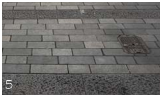
SPECIAL PAVING TO SPAN ACROSS BOTH LOTS AT FUTURE C STREET
