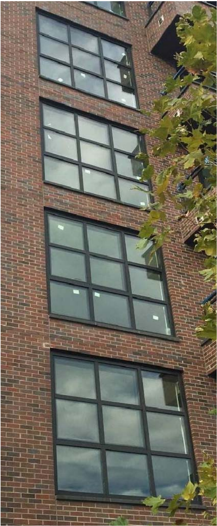
05 FRAME SIZE: 108 X 84 W-2500 STD CLAD MULL AURALAST PINE, CASEMENT/AWNING PRODUCT, BLACK EXTERIOR, PAINTED WHITE INTERIOR FRAME/SASH, NAIL FINISH(STANDARD), COLOR MATCH METAL DRIP CAP, 3 WIDE. 3 HIGH, 6 9/16 JAMB, INSULATED LOW-E 366 ANNEALED GLASS, NO PRESERVE FILM, ARGON FILLED
