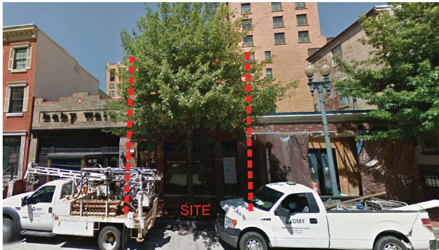
VIEW 2 - 9TH STREET EXISTING CONDITION
