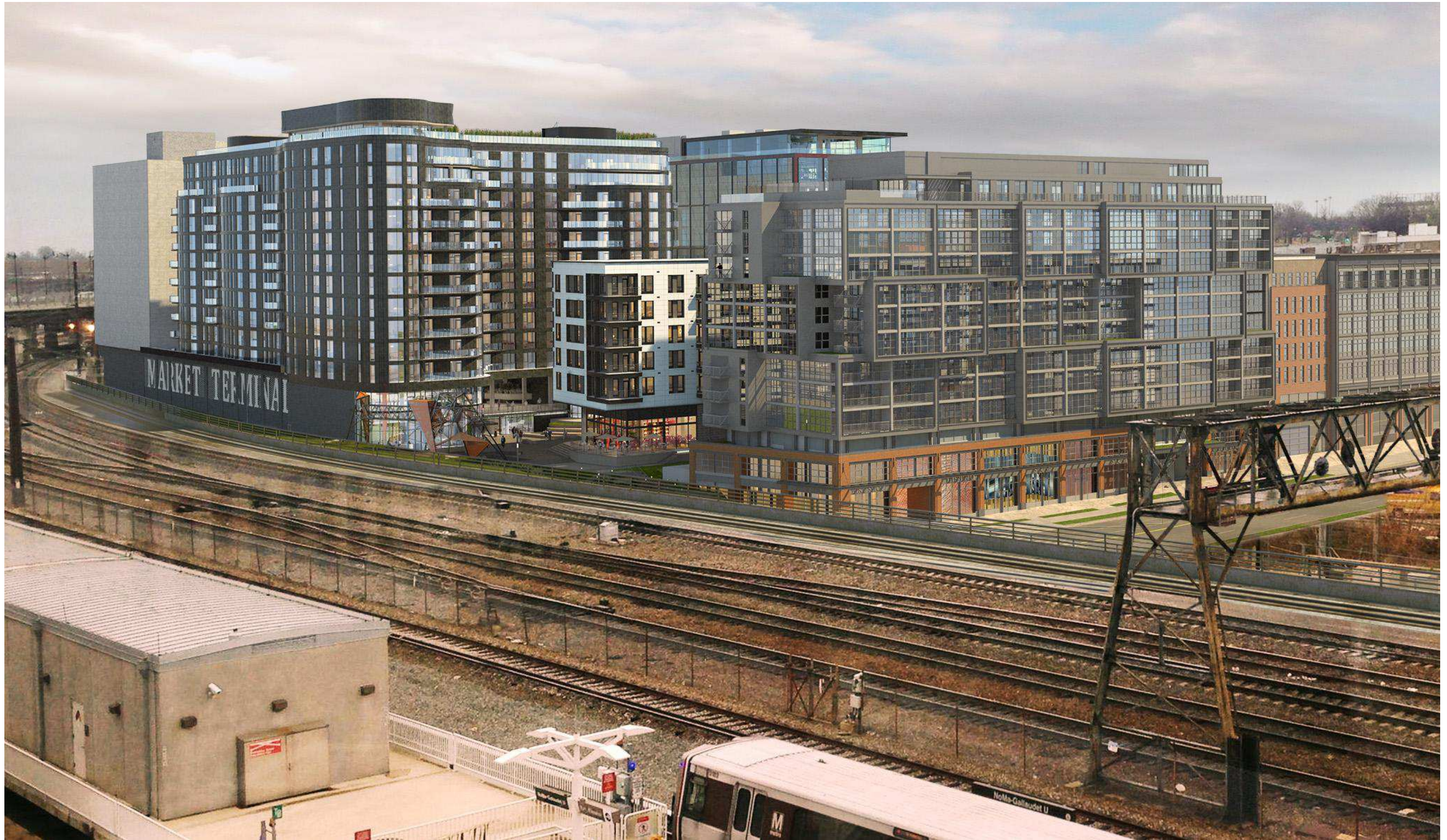
VIEW FROM LOOKING SOUTH-EAST OVER TRAIN TRACKS
