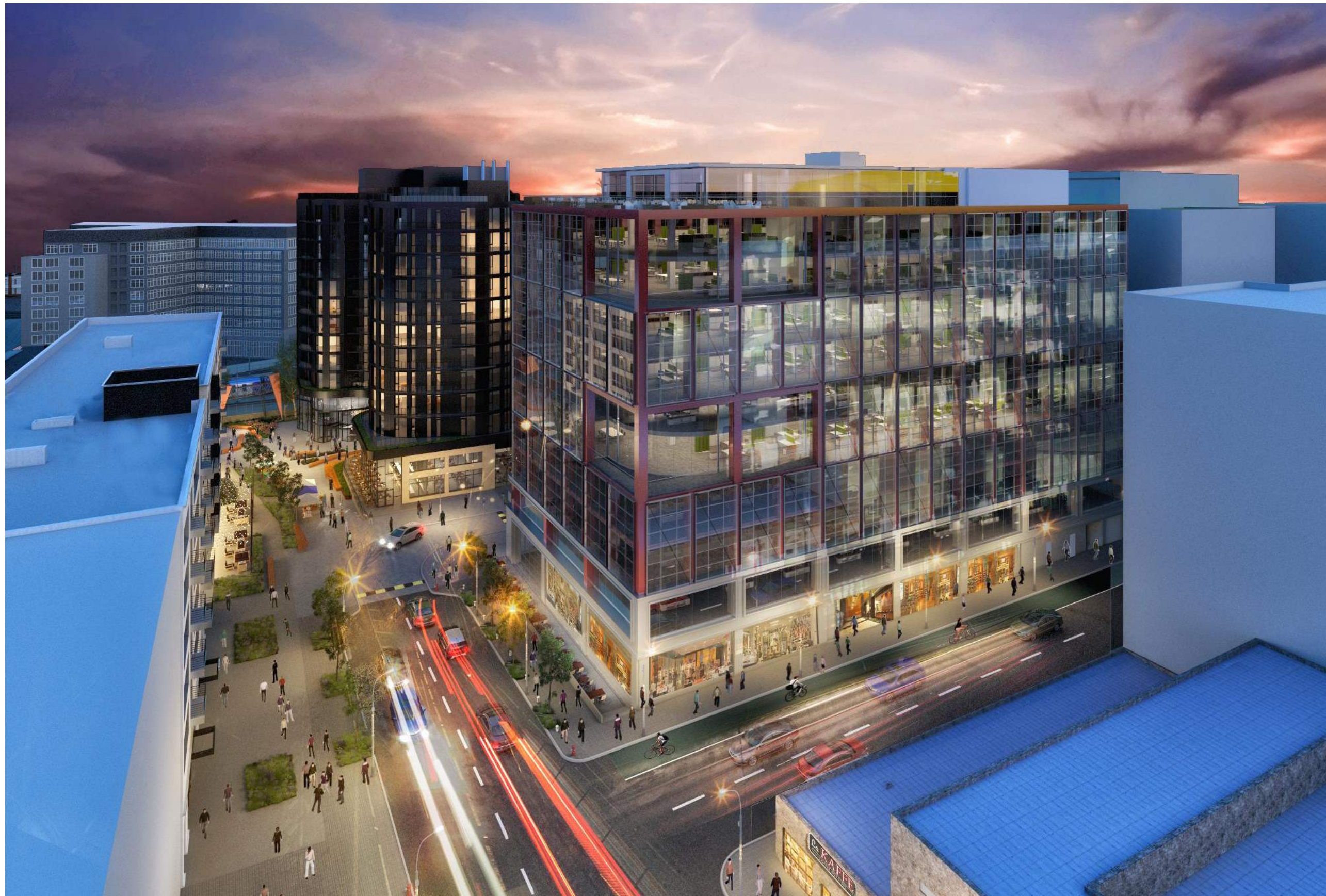
VIEW LOOKING WEST ON MORSE ST NE
